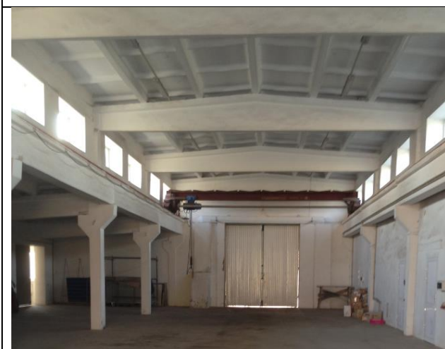
Picture 11 Manufacturing facility № 1 and the loading crane
